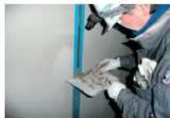
PRS joint filling method
