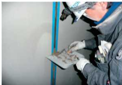
PRS joint filling method
