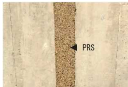
PRS joint filling method
