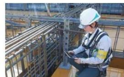
Bar arrangement inspection using tablets
