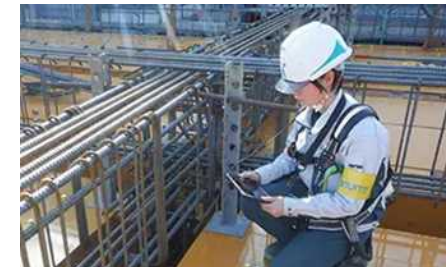
Bar arrangement inspection using tablets
