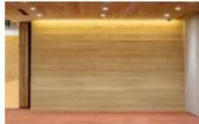
Soil wall construction system
