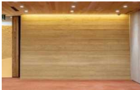
Soil wall construction system
