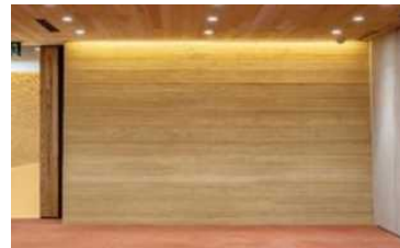
Soil wall construction system
