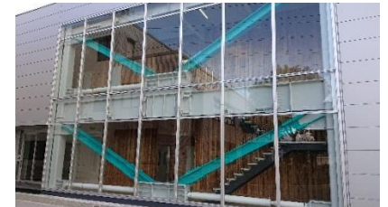
2 Seismic dampers in additional buildings
