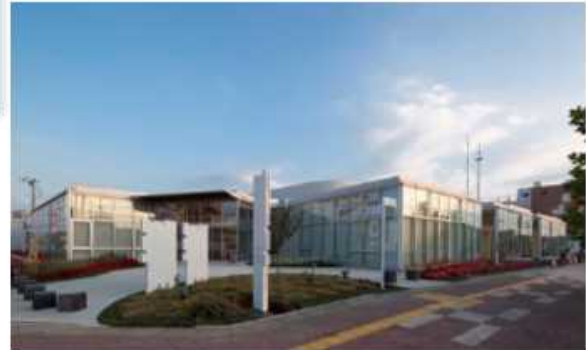
"Cosmos Fukiage-kan" Winner of the 17th Public Building Construction Award for Excellence
