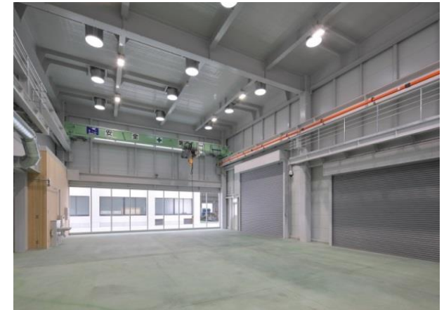
Expansion Building and Multipurpose Experimental Space Using Natural Light Illumination
