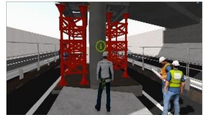
High-speed cross-bridge pier repair
