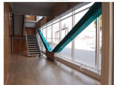
Quake-absorbing dampers
